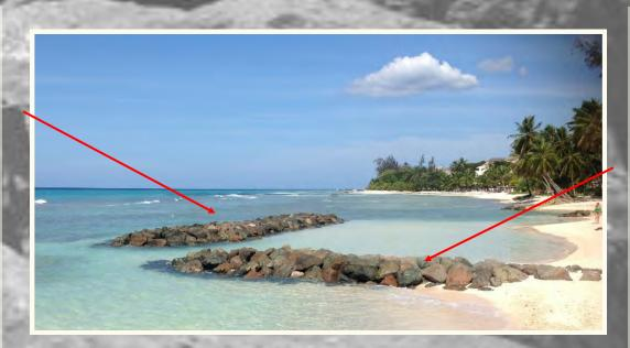
Groynes are lines of boulders laid in the sea, constructed perpendicular to the beach.
