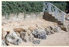
Revetments are piles of boulders or gabions (wire baskets filled with rocks), placed at the base of coastal structures to diffuse wave energy. They may be seasonally covered with a thin layer of sand, but this is usually too shallow for a turtle to dig into
